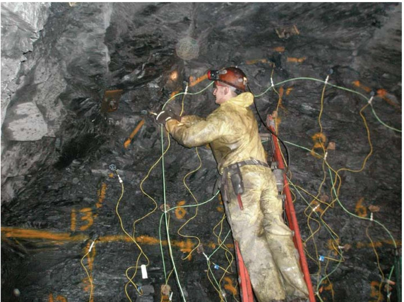
Figure 7. Tying up at heading.
