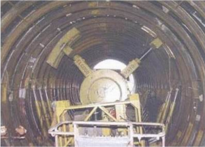
Figure 2: Expanded steel sets reshape the tunnel geometry.
