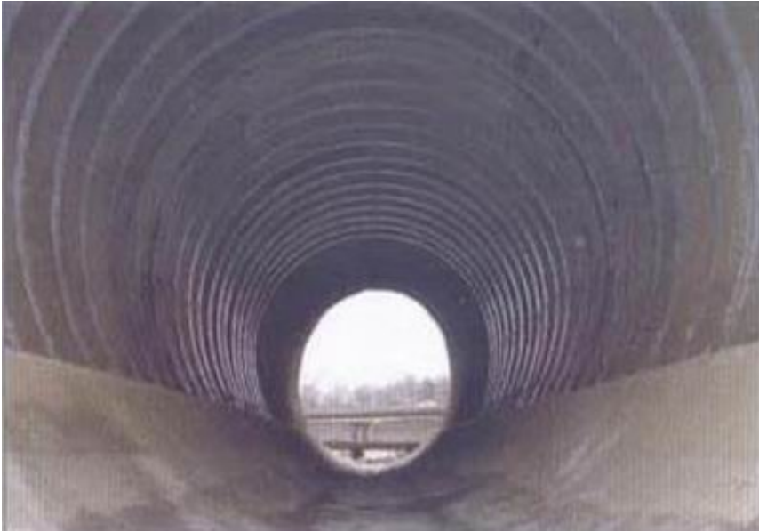
Figure 3: Repaired culverts relined with fiber-reinforced shotcrete.
