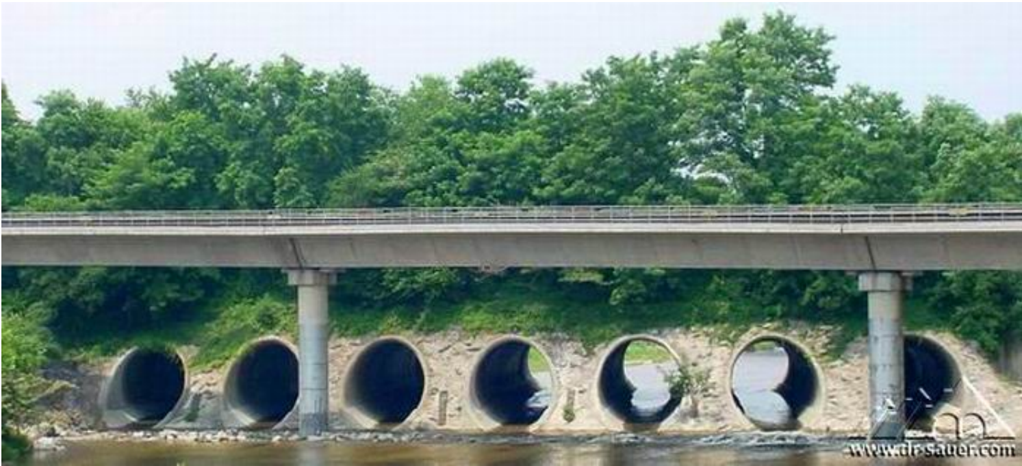
Figure 4: Finished Cameron Run culverts.
