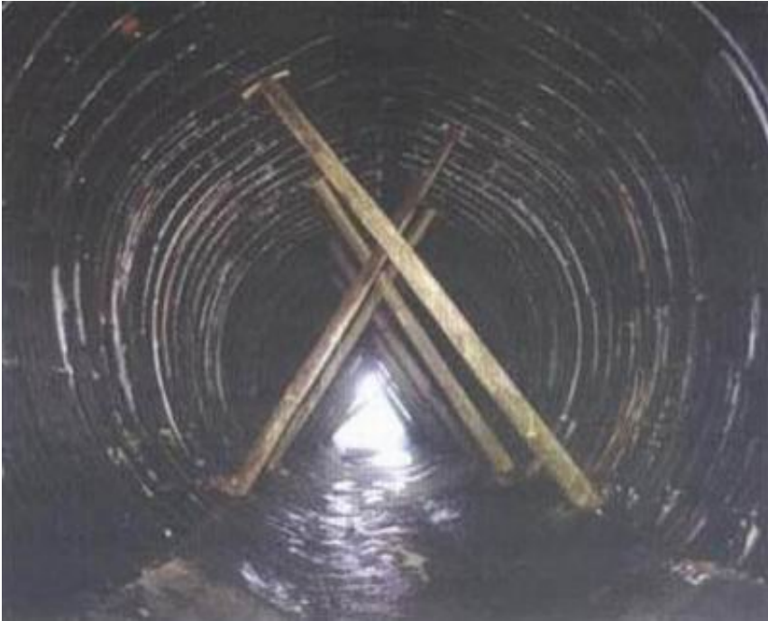
Figure 1: Props supported the liner plates of the old culverts.
